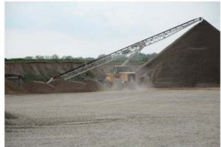
PROCESSING AREA IN EXISTING PIT
