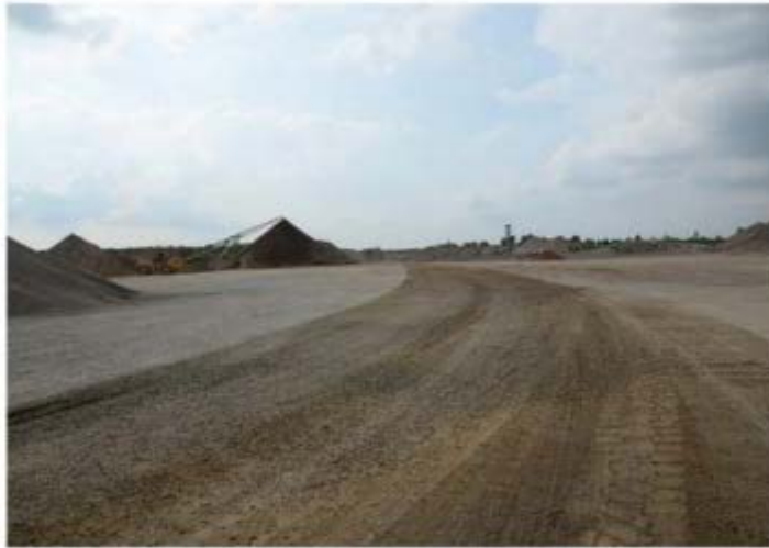
HAUL ROAD IN EXISTING PIT TREATED WITH DUST SUPPRESSANT
